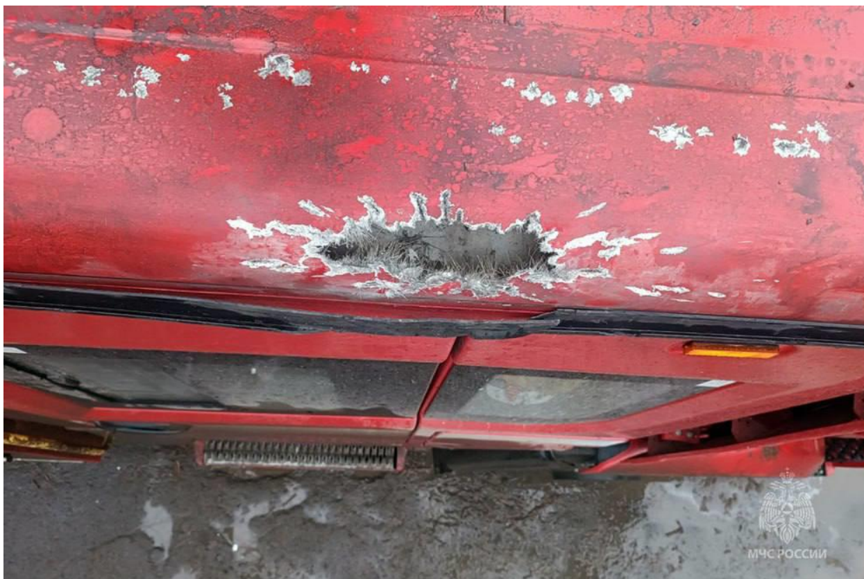
Fig. 14 – Damage to a fire truck from the explosion of a high-pressure explosive device dropped by a UkrainianUCAV.
