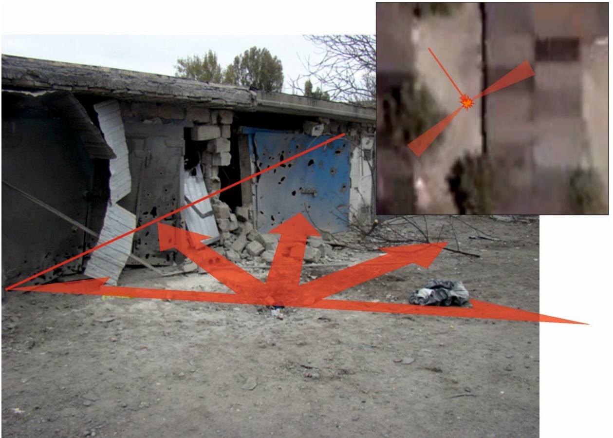
Fig. 15 –Projectile explosion diagram in case of shell hit 1.
