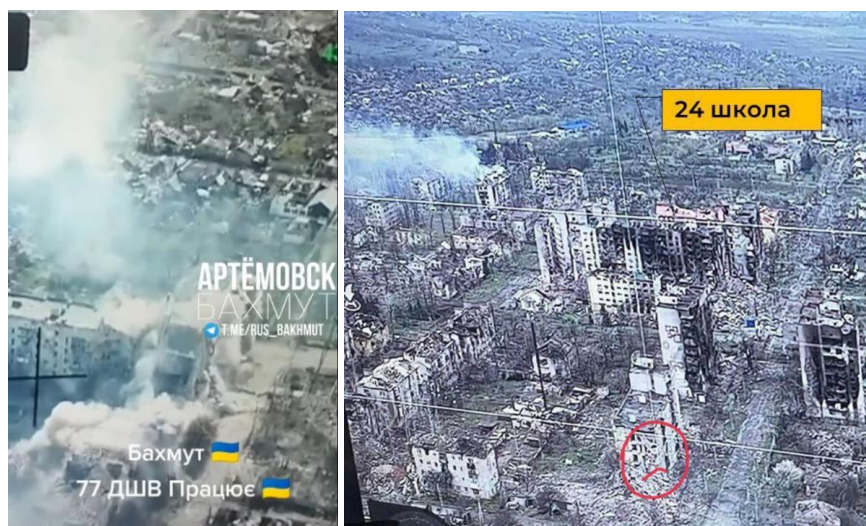
Fig. 13 – “7-5-7” Residential building at 36 Levanevsky Str.: on the left – the moment of the building demolition, on the right – consequences 25 of the building demolition.
