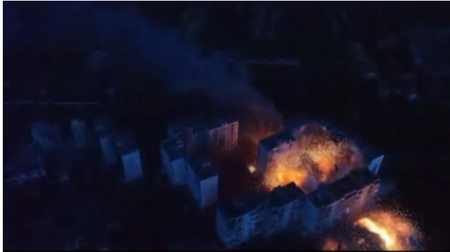
Fig. 6 – Demolition of a multi-storey residential building at 105, Tchaikovsky Str.
