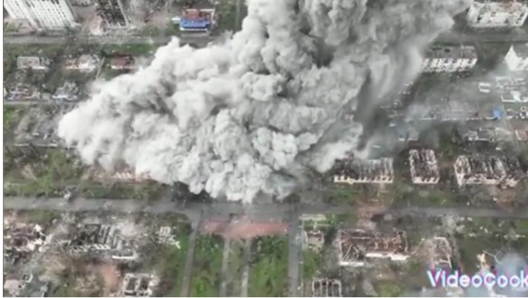
Fig. 3 – Demolition of the House of Culture at 23A, Pobedy Street.
