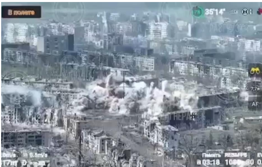
Fig. 9 – Demolition of the a five-storey residential building at 1, 60 Years of the USSR Formation Street.
