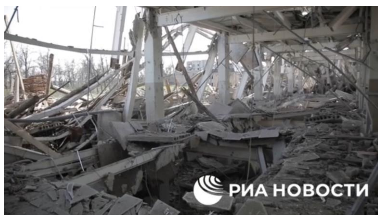
Fig. 5 Consequences of the demolition by Ukrainian military personnel of the building of the former sewing factory “The 8th of March” at 16 Rozhdestvenskaya Str.
