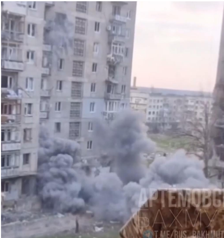
Fig. 8 – An unsuccessful attempt at a controlled demolition of a multi-storey residential building at 113, Yubileinaya Str.
