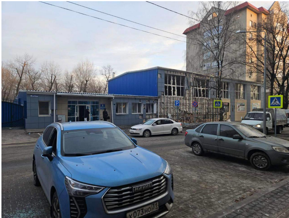
Fig. 2 - Shell hit in close proximity to the Dynamo stadium. 13
