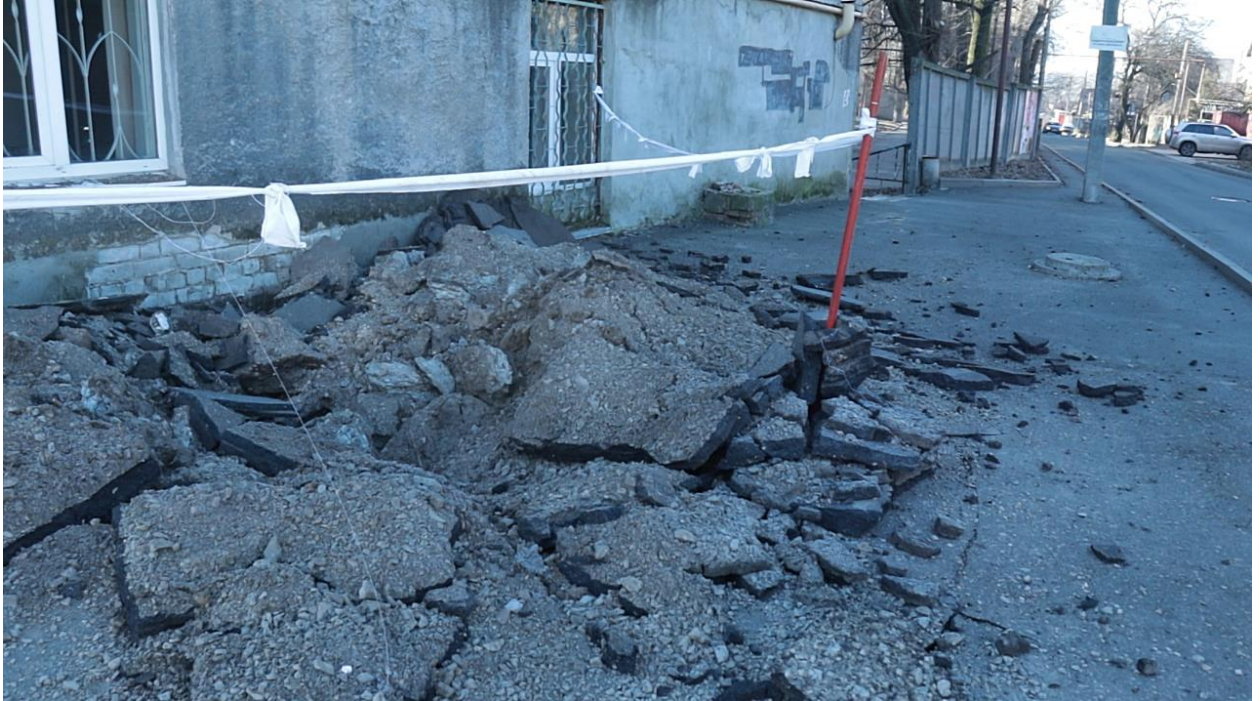
Fig. 16 – A camouflet near the dormitory of the M. Gorky DoNMU after the shelling on December 19, 2022
