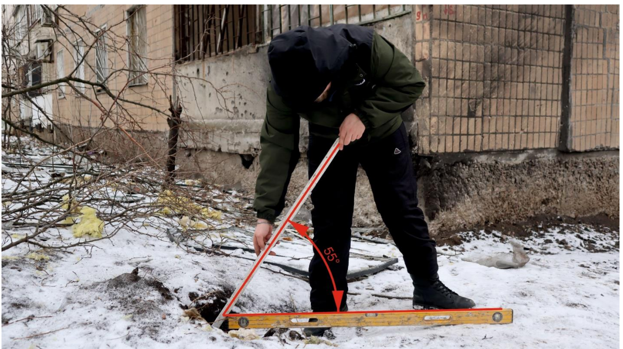
Fig. 52 – Determining the angle of impact with a horizontal surface at the site of shell hit 11 of December 19, 2022
