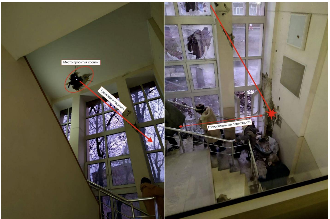
Fig. 43 – A projectile fall line at the site of shell hit 2 of December 11, 2022
