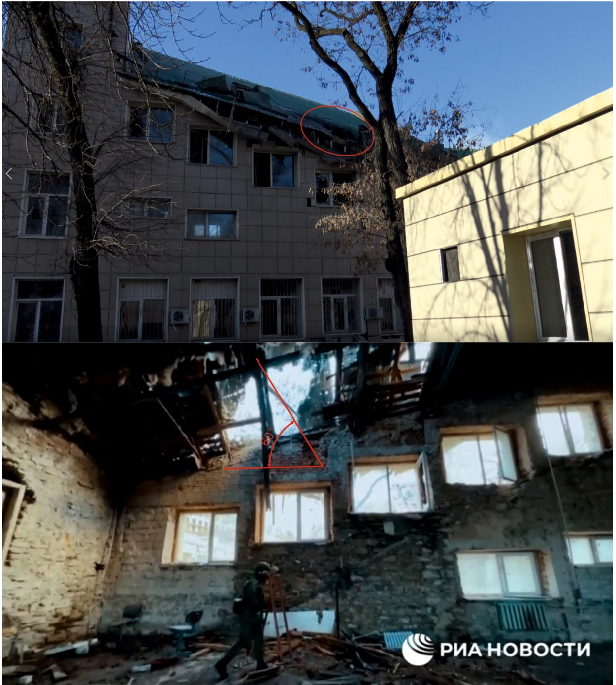
Fig. 46 – Determining the angle of impact with a horizontal surface at the site of shell hit 4 of December 18, 2022 (photo above: exterior view of the DoCTMA building No. 7; photo below 62 : interior view of the building No. 7).
