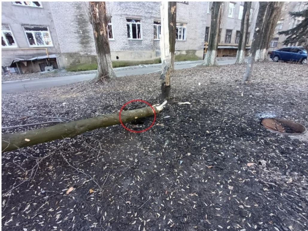
Fig. 17 – A crater from a projectile in the territory of the M. Gorky DoNMU between the sports and recreation complex and building No. 1 after the shelling on December 19, 2022
