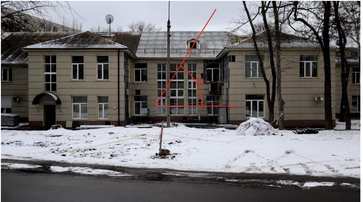
Fig. 44 – Determining the angle of impact with a horizontal surface at the site of shell hit 2 of December 11, 2022
