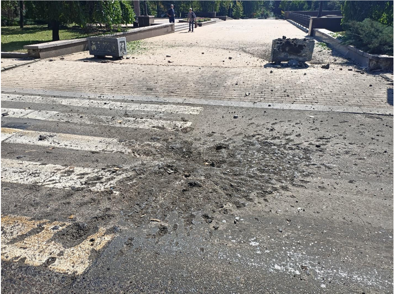
Fig. 2 - Shell hit 1 located in the central alley of Pushkina Boulevard.
