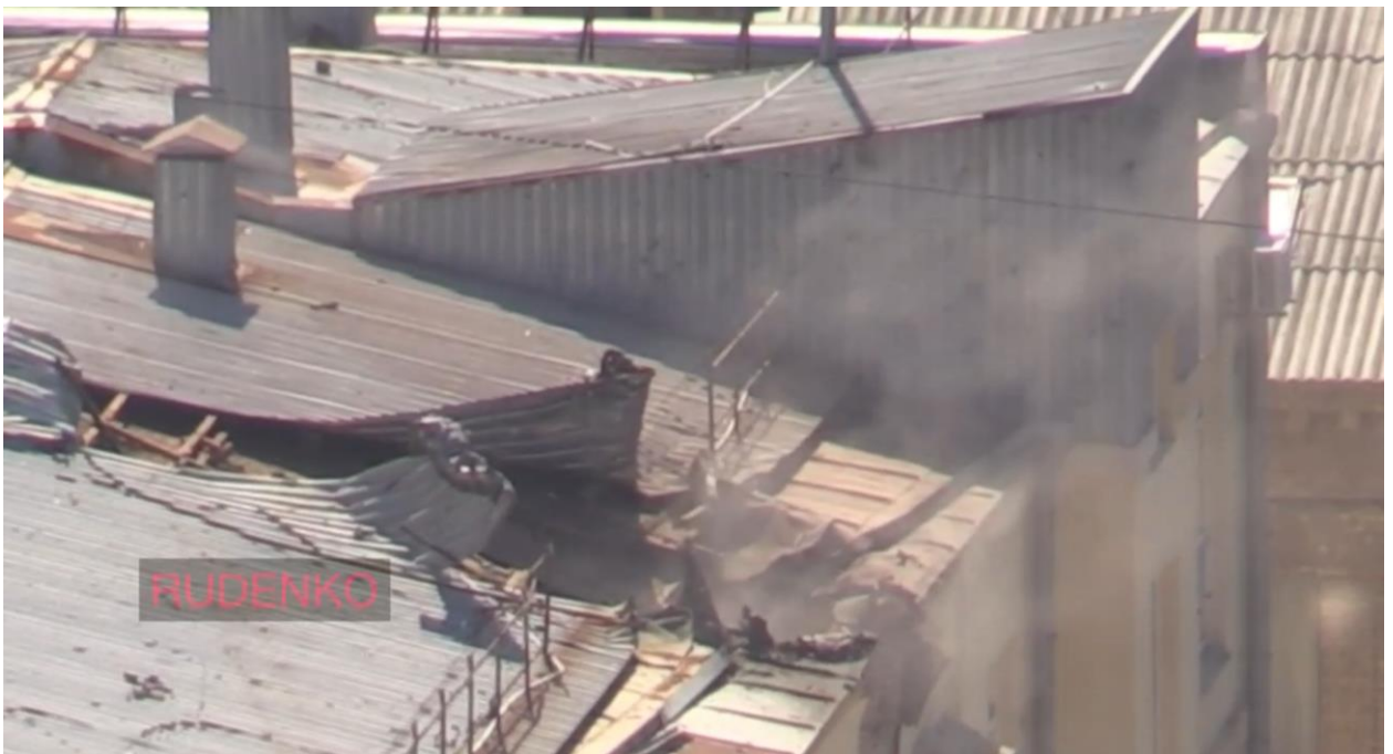
Fig. 8 - Shell hit 7 in the roof of the Donbass Post building
