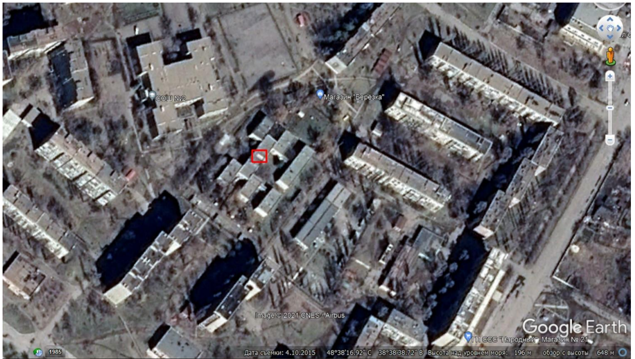
Fig. 5 – The trail of a shell hit 2 on the kindergarten roof on the satellite image dated 10.04.2015.
