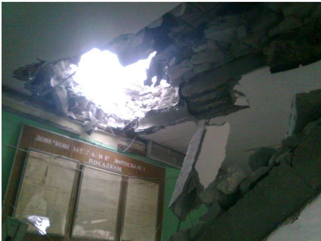
Fig. 16 – The through hole in the roof of the technical college damaged as a result of shell hit 7 35 .
