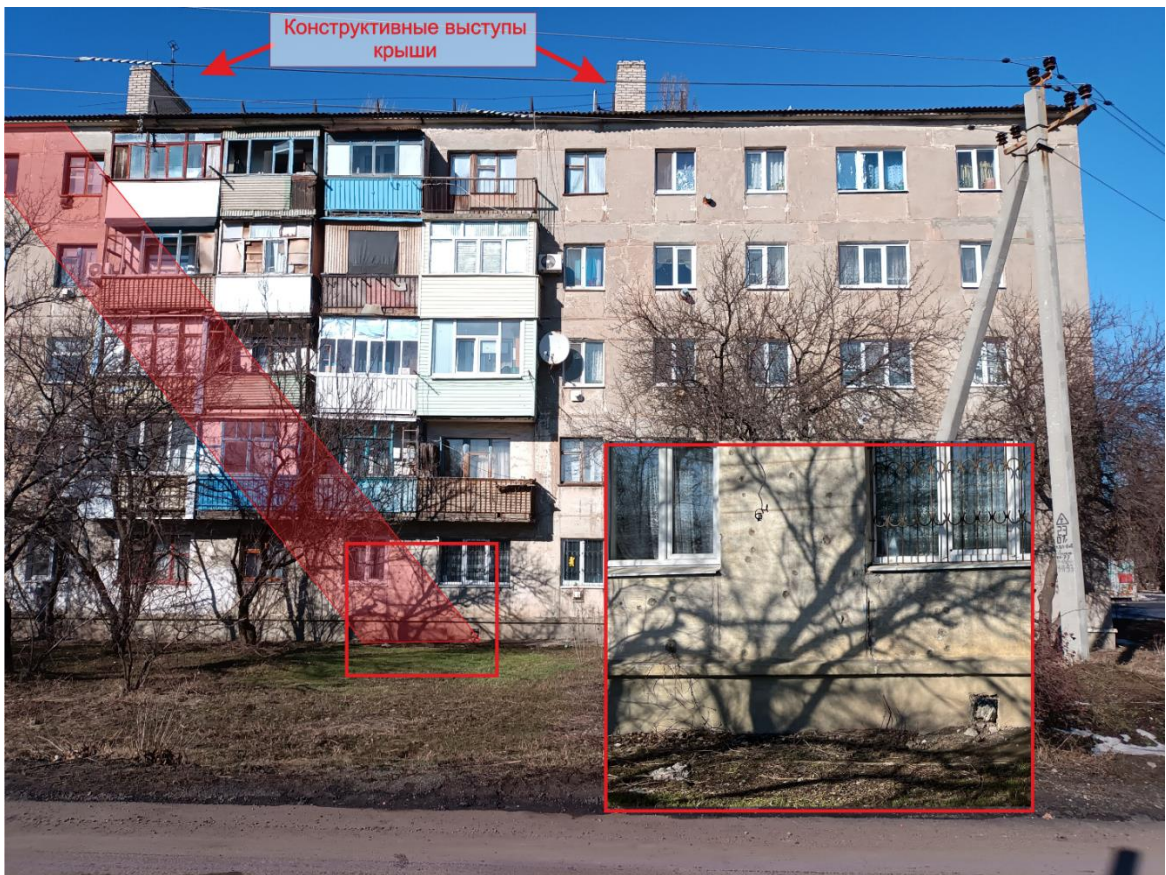
Fig. 37 - The line of the main scatter of fragments on the residential building as a result of shell hit 8.
