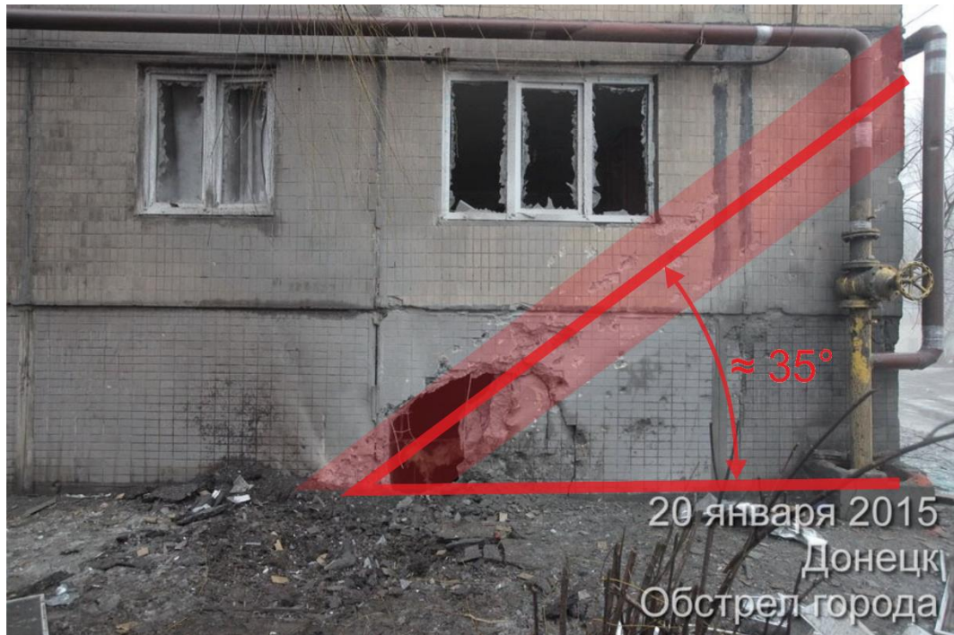
Fig. 30 – Fragment scattering angle (shell hit 3) 58 .
