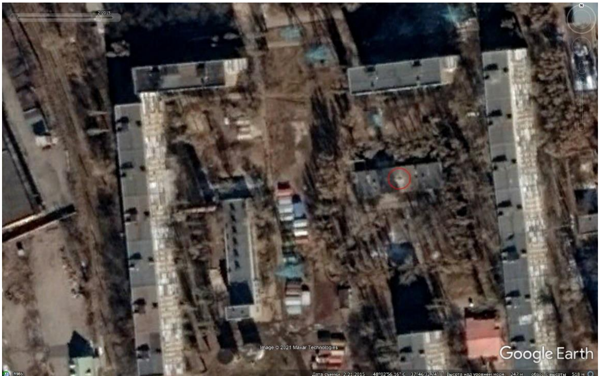
Fig. 4 – The trail of a shell hit on the roof of Nursery School No. 204 on the satellite image dated 02.21.2015
