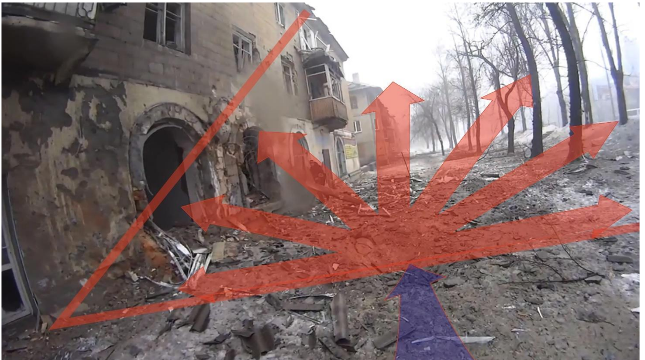
Fig. 27 - The fragment scattering pattern at the shell hit 7.
