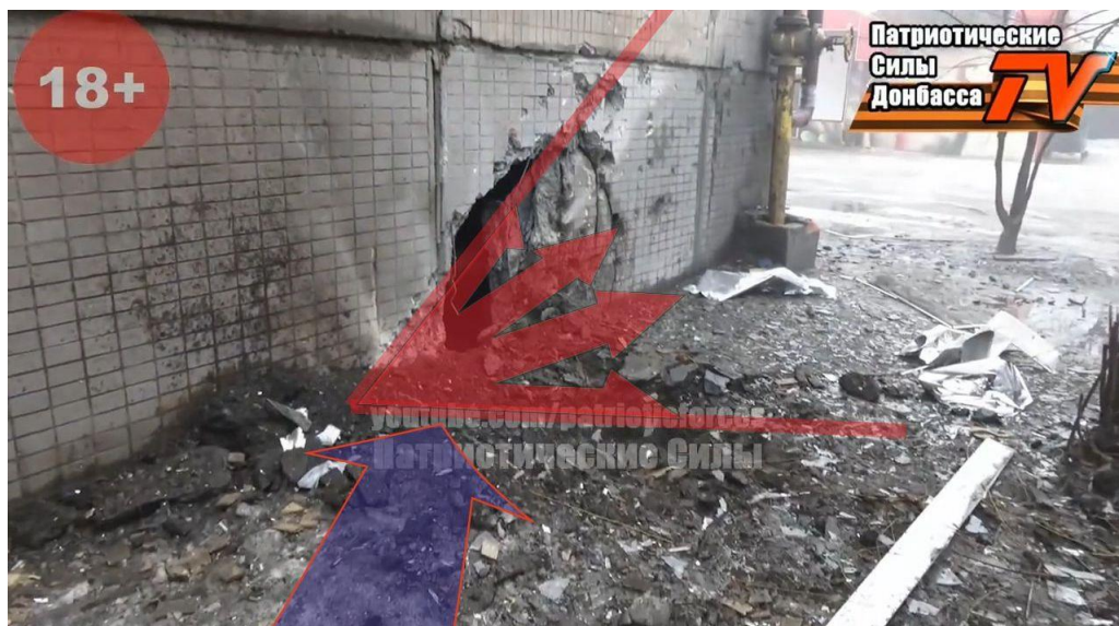
Fig. 25 – The fragment scattering pattern at the shell hit 3.
