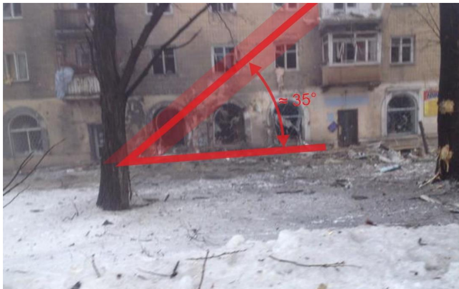
Fig. 31 - Fragment scattering angle (shell hit 7) 59 .
