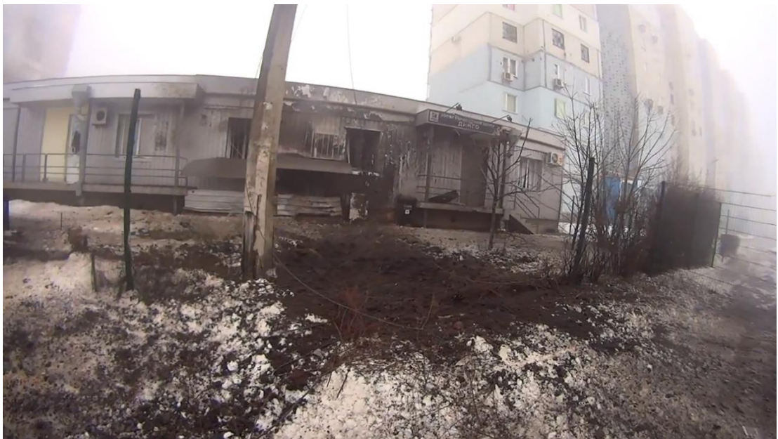
Fig. 9 – An artillery shell explosion crater on the lawn next to a one-story building located at 20A, Politboitsov St. 45 .
