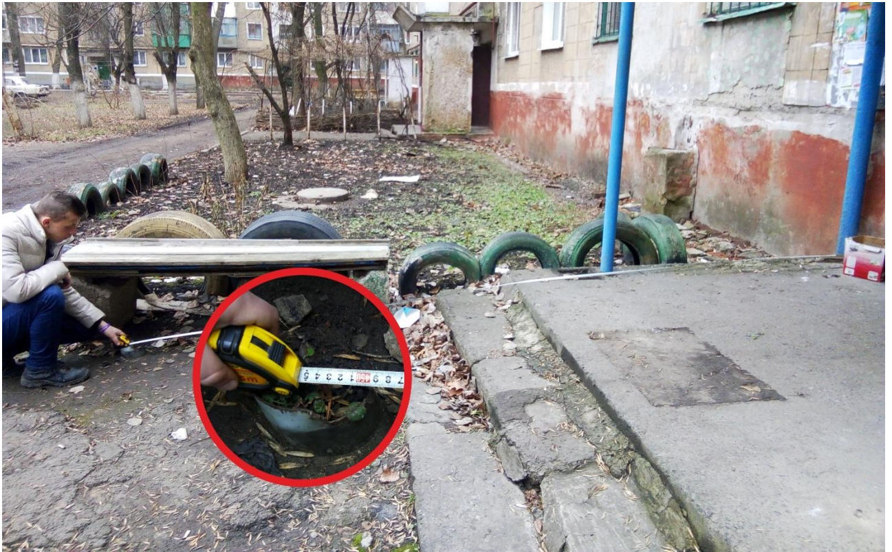
Fig. 19 – Measuring the distance from the wall of the residential building to the center of the crater from the explosion at the shell hit 5 (14.12.2021).
