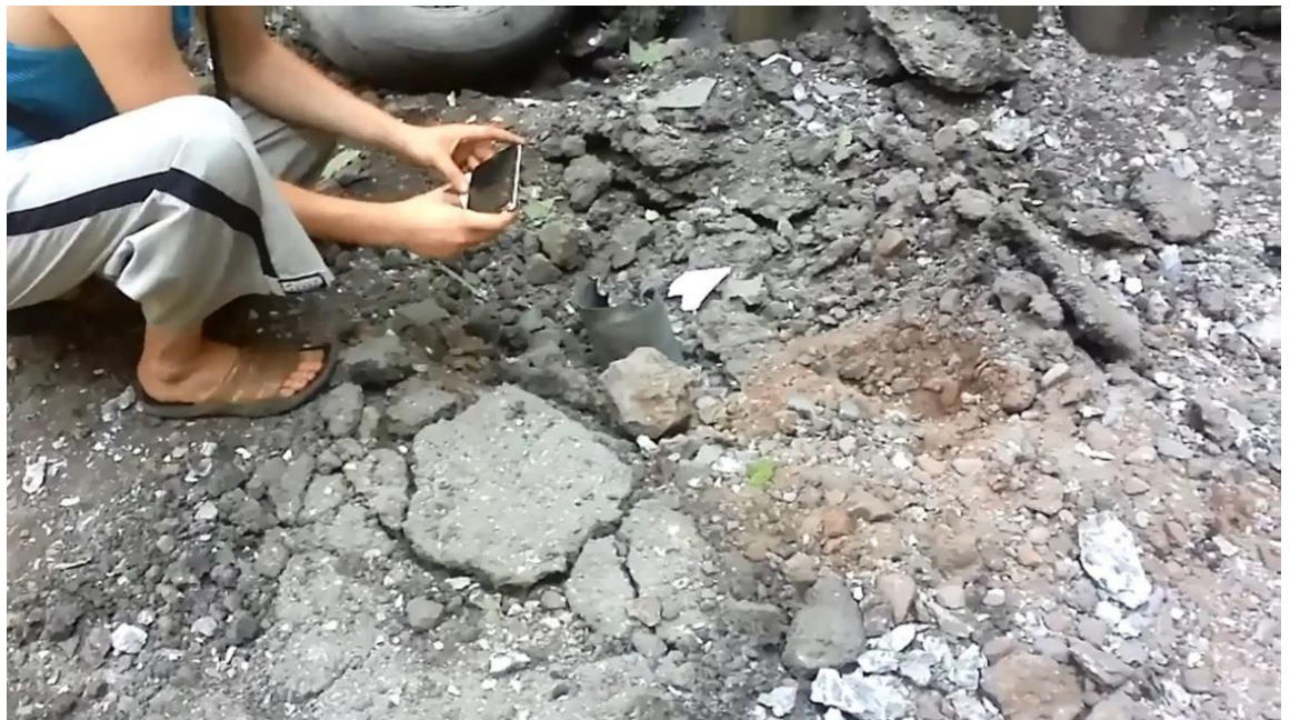
Fig. 9 - Debris of the projectile missile part a few meters away from the third entrance hall of the residential building at 4, Cosmonaut Volkov St., Horlivka 22 .
