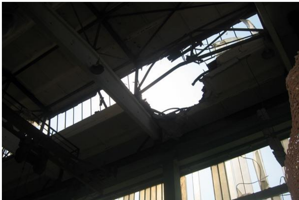
Fig. 15 – A hole in the roof of the DonNTU ESR laboratory building, formed as a result of shell hit 7 44 .
