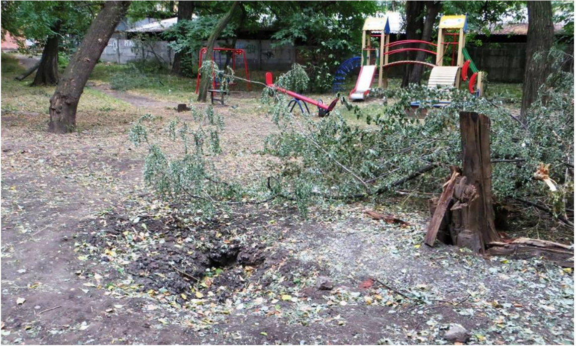
Fig. 6 – Shell hit (2) in the ground surface about 15 meters south-east of the south-western corner of building No. 58B in Artyom Str 35 .
