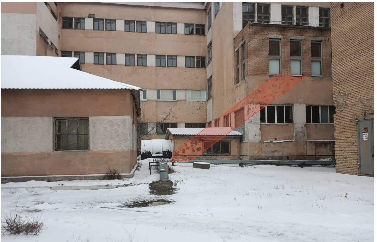
Fig. 27 – Traces from the main scatter of fragments on the wall to the east of shell hit 8 (photo from January 24, 2022).
