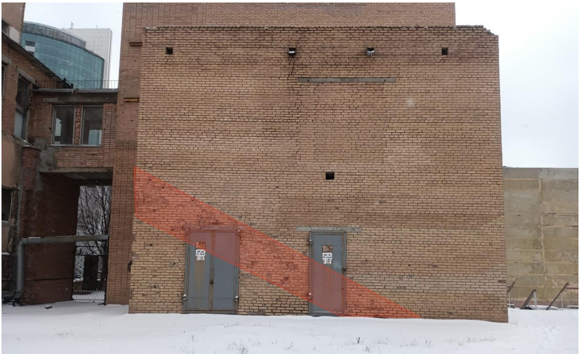
Fig. 28 – Traces from the main scatter of fragments on the wall to the south of shell hit 8 (photo from January 24, 2022).
